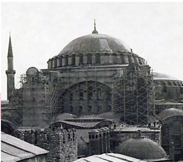
CTA_S103_A03_phg_01: Northern façade of Saint Sophia during restoration, 1956, S103, A03, phg01
